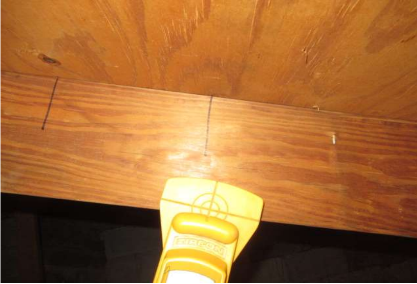
Nail location verified
