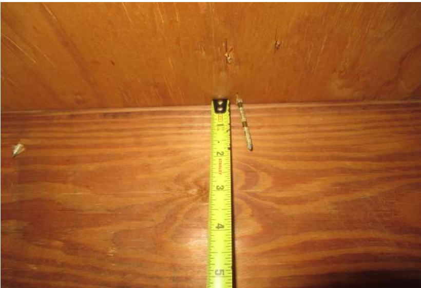
8d nails verified
